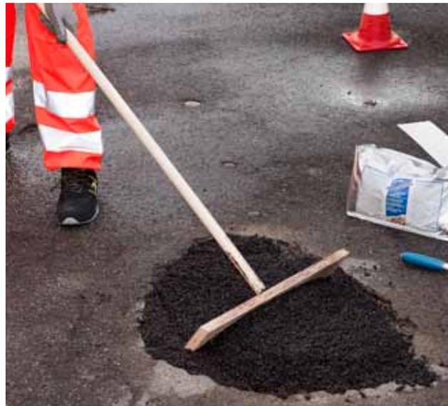
2. Applying and spreading **Mape-Asphalt Repair 0/8**
