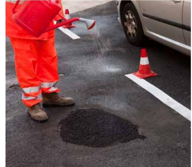
3. Wetting the surface of **Mape-Asphalt Repair 0/8**
