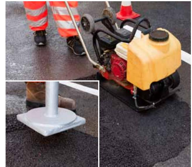
4. Manual or mechanical compacting of **Mape-Asphalt Repair 0/8**
